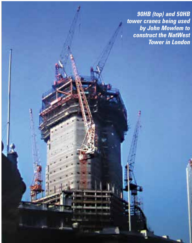
The HB cranes could self-install additional tower sections directly through the slew ring
