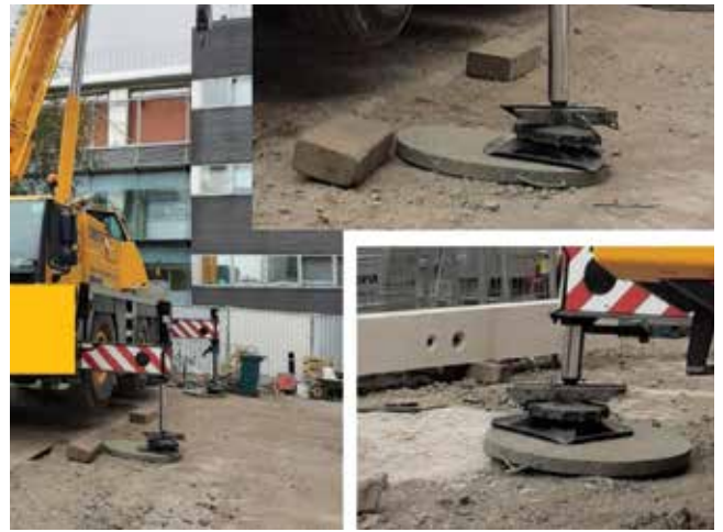
Some of the real life examples found on site
