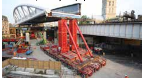
Engineered Rigging's rental fleet included a 2,200 ton jack up system
