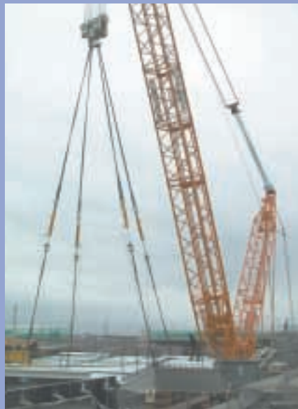
Bridge segments are positioned using Enerpac's SyncHoist system.
