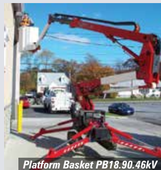
Platform Basket PB18.90.46kV
