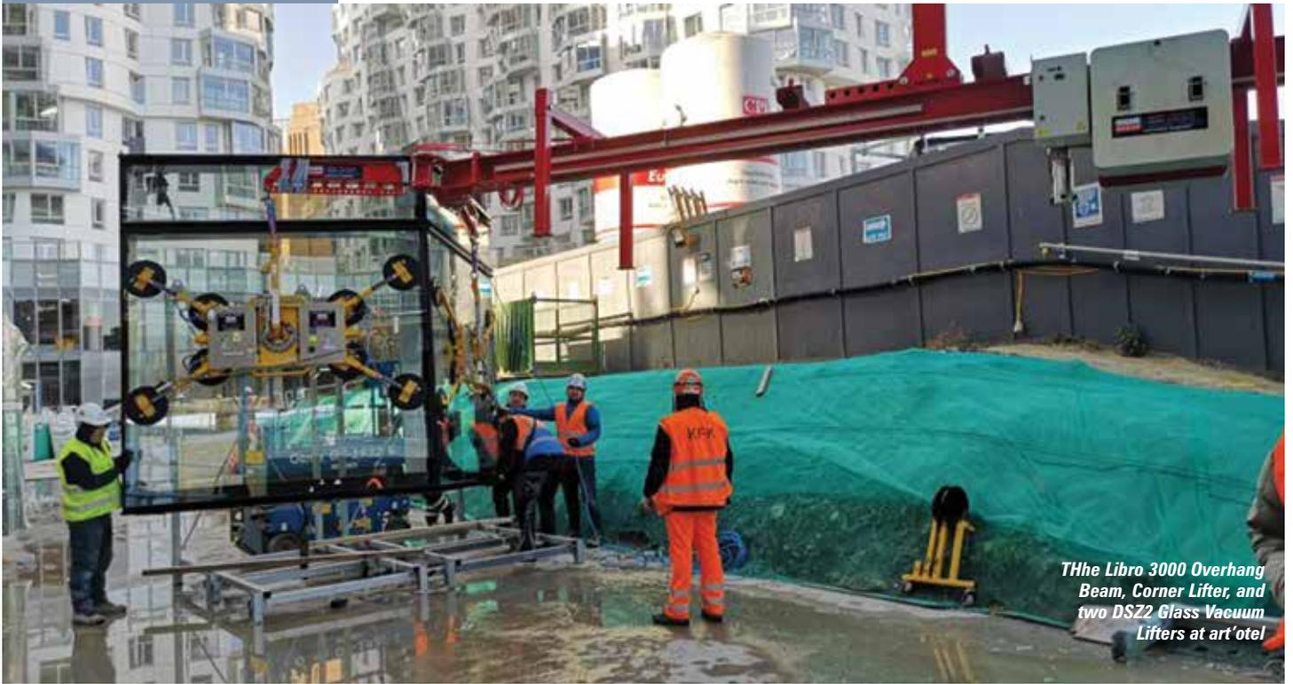
*The Libro 3000 Overhang Beam, Corner Lifter, and two DSZ2 Glass Vacuum Lifters at art'otel*
