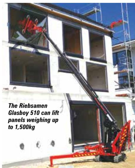
The Riebsamen Glasboy 510 can lift panels weighing up to 1,500kg
