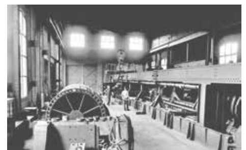
The massive Avery test machine in the Test House that is still going strong today was commissioned to test girder beams up to 1,250 tonnes Sydney Harbour Bridge
