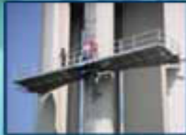
Malmqvist High Climber MA-2000, renovation work in Sweden.
