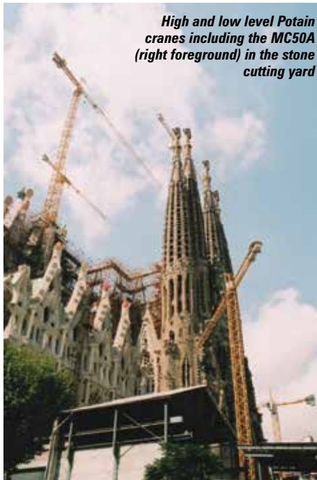
The ballasted base of the Potain MD235A was erected 54 metres up on the roof
