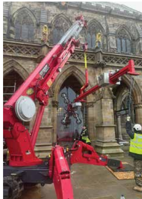
The Grade One listed Rochdale Town Hall installation required a Unic URW-706 spider crane with Libro 2500B overhang beam and GL-UMC1200 glass manipulating head
