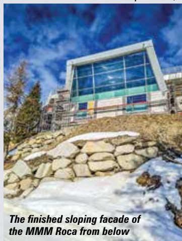
A pane is lifted into the sloping façade
