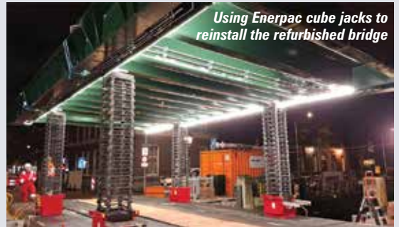
Enerpac cube jacks raise the bridge ready to be rotated on the slew ring
