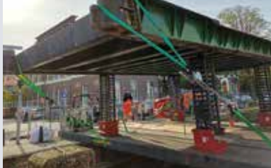
Enerpac cube jacks raise the bridge ready to be rotated on the slew ring
