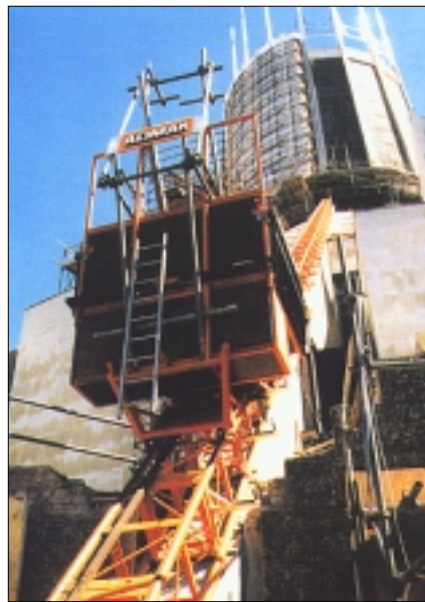
Hoist-it's Alimak goods hoist at Liverpool's Catholic Cathedral
