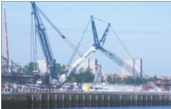
Baldwin's Liebherr LTM-11000D mobile crane was deployed, after dismissing the use of helicopters or barge mounted cranes
