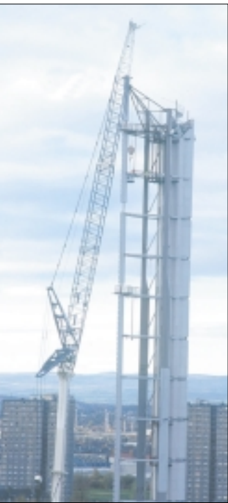
Baldwin's Liebherr LTM-11000D mobile crane was deployed, after dismissing the use of helicopters or barge mounted cranes
