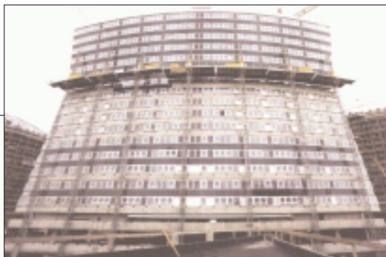
HEK has no problems with sharp corners and curves (seen here in Austria)
