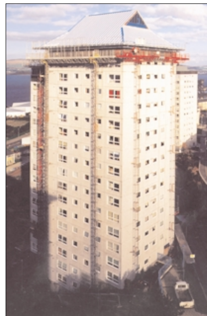
Mastclimbers used to install new roofs on tower block in Greenock
