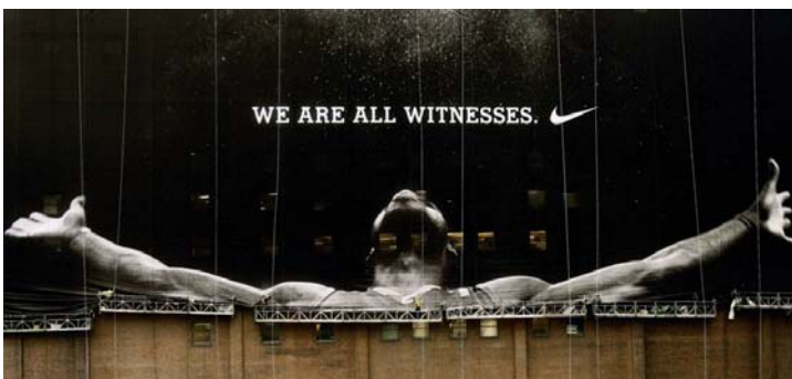
The Spider division of SafeWorks recently used seven suspended platforms to take down the huge 10 storey Nike banner advert in Cleveland.
